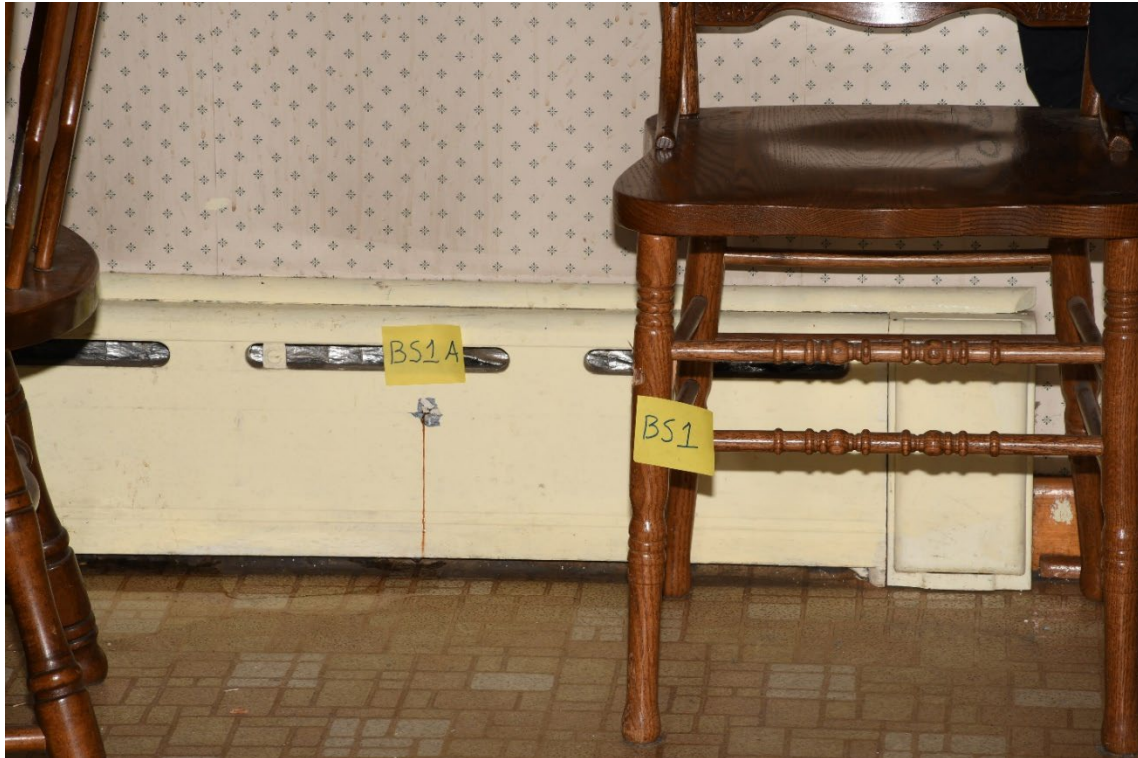
Damaged Chair and Wall
